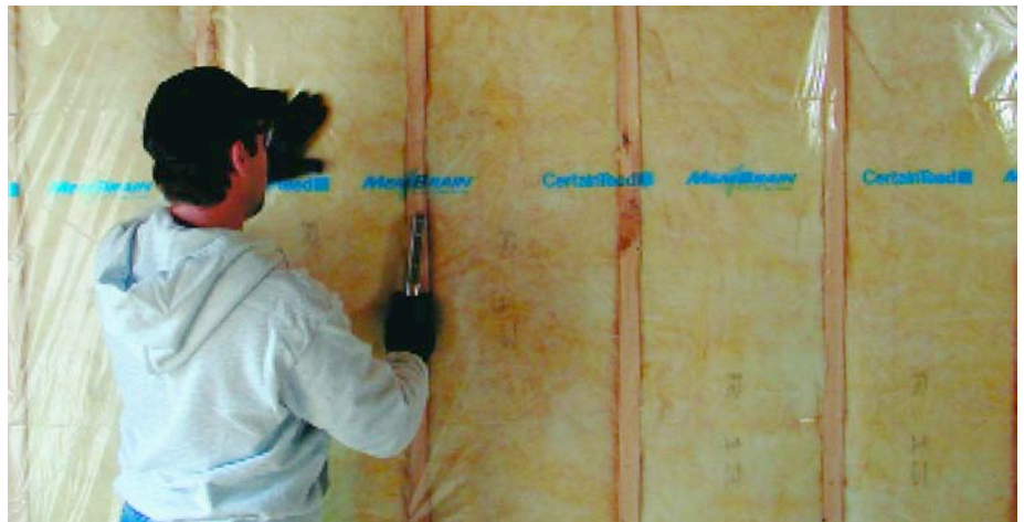
MemBrain Protects: When the relative humidity in insulated cavities is low, molecular-scale pores close and work as a vapor retarder.
